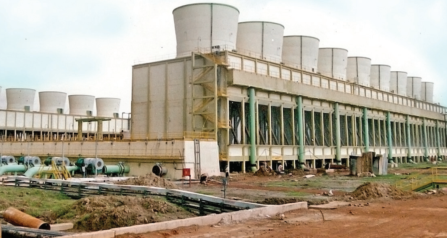
An under-construction cooling tower at Haldia
