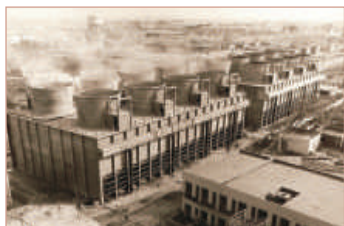
Mechanical Draft Cooling Towers
