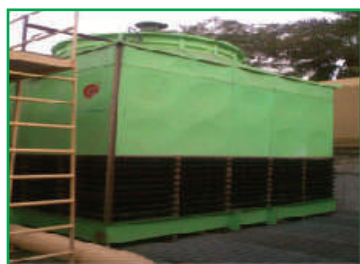
Package FRP Cooling Tower
