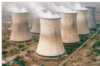
Natural Draft Cooling Towers
